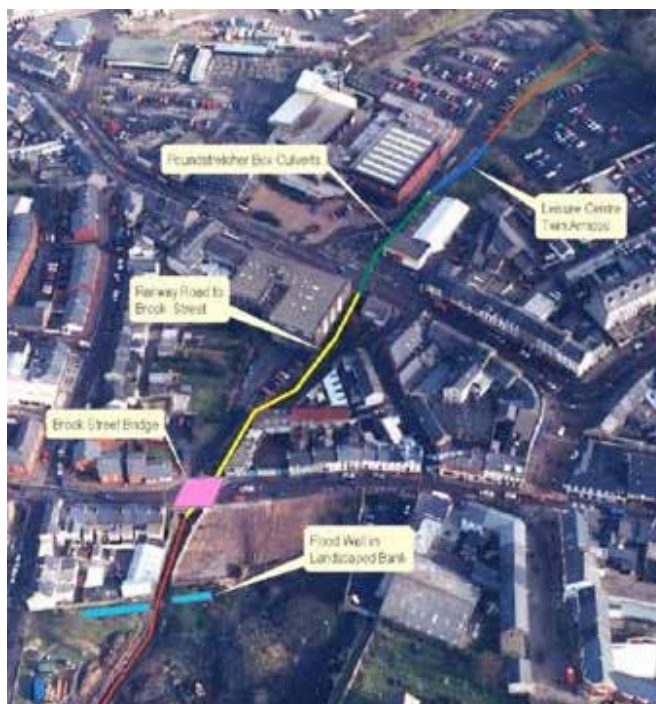
Overview of Lodge Burn Flood Alleviation Scheme
