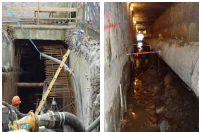
Poundstretcher culvert during refurbishment works (these are not services within the culvert but are bracing structure and the flow bypass pipe)
